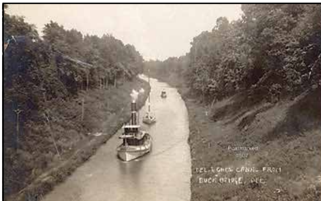
Figure 2 The C & D Canal in 1907 (Cecil)
